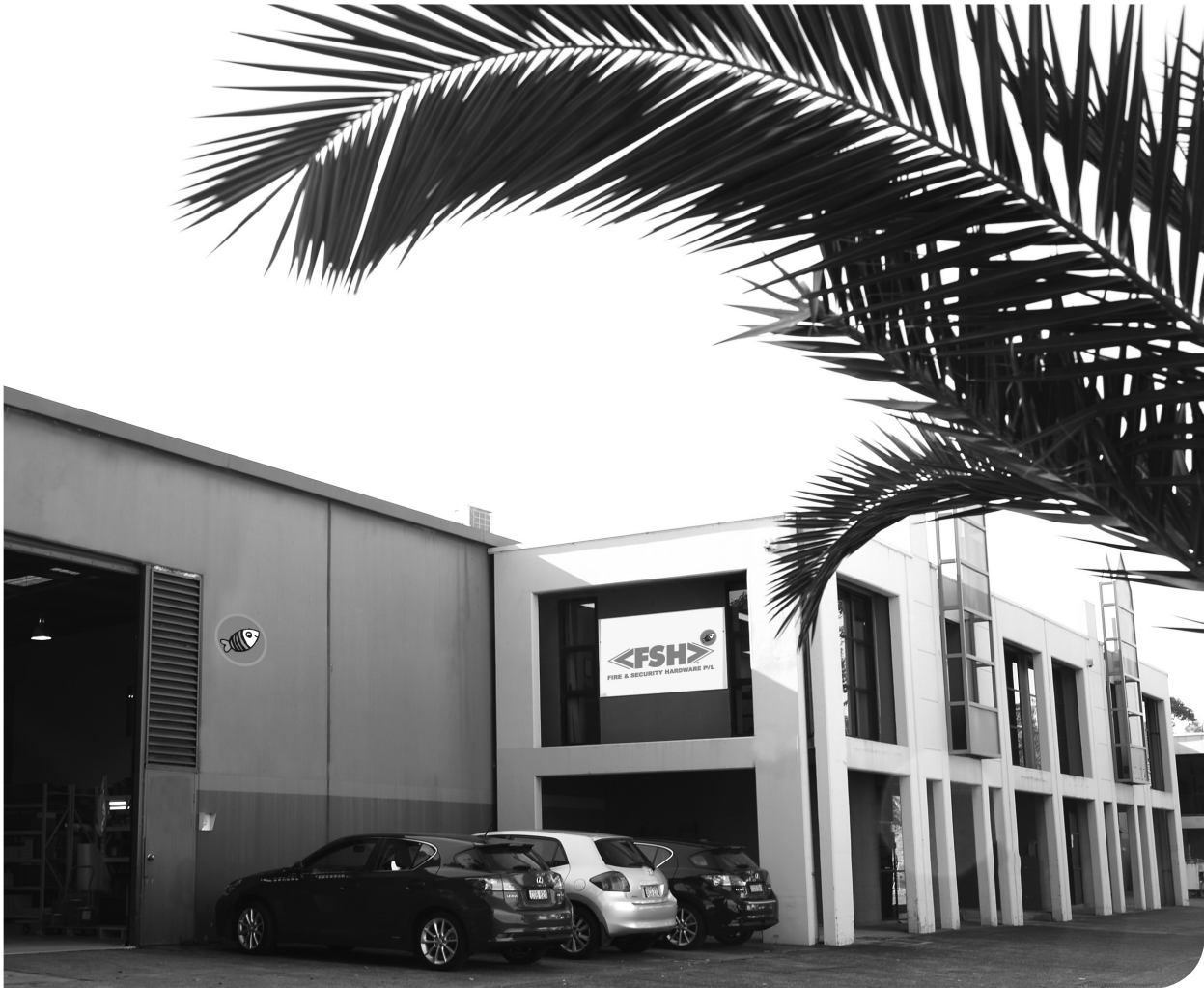
FSH HEADQUARTER | MATRAVILLE NSW
